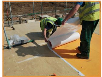
**Step 3.** Working in pairs, roll out the mat progressively whilst peeling away the release paper. For large areas, use a dry roller to smooth out.
