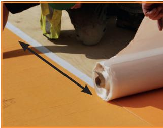
**Step 4.** Ensure that each new length of mat overlaps on the white strip to bond and seal the previous length.
