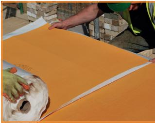
**Step 2.** Attach the adhesive side to the surface that needs to be protected.
