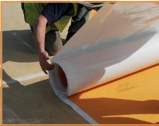
**Step 1.** Peel away approximately 12 inches of release paper from the Stickymat adhesive layer.
