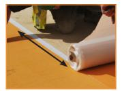
**Step 4.** Ensure that each new length of mat overlaps on the white strip to bond and seal the previous length.
