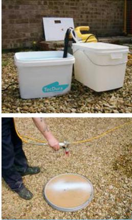
**2.** Point the nozzle at the area you wish to protect and hold the spray gun 300-400 mm from the substrate. Use the TecDura shield to prevent overspray.
