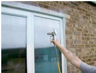
**4.** Release the trigger at the end of each stroke. Then depress the trigger and overlap the previous pass by about 50%. Continue in this fashion for consistent coverage working down the substrate.
