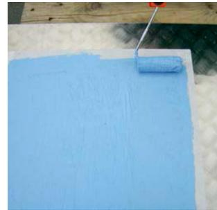
**3.** Use a wet film gauge to check the coatings wet film thickness; make sure this is the same minimum WFT as stated in the product's Technical data sheet (TDS).
